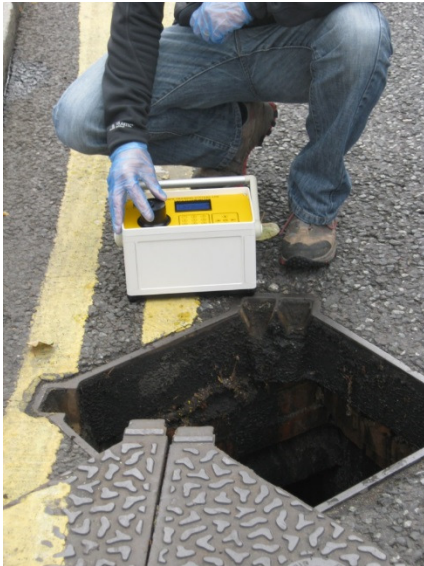
Misconnection monitoring at the road side
